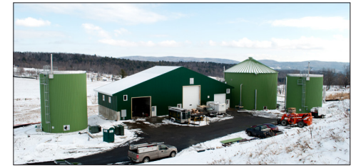
"Big Bertha" is Vermont Tech's community anaerobic digester, capable of generating 8,800 kWh per day.
